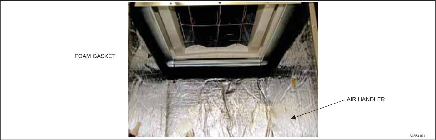
FIGURE 4: Gasket Location
